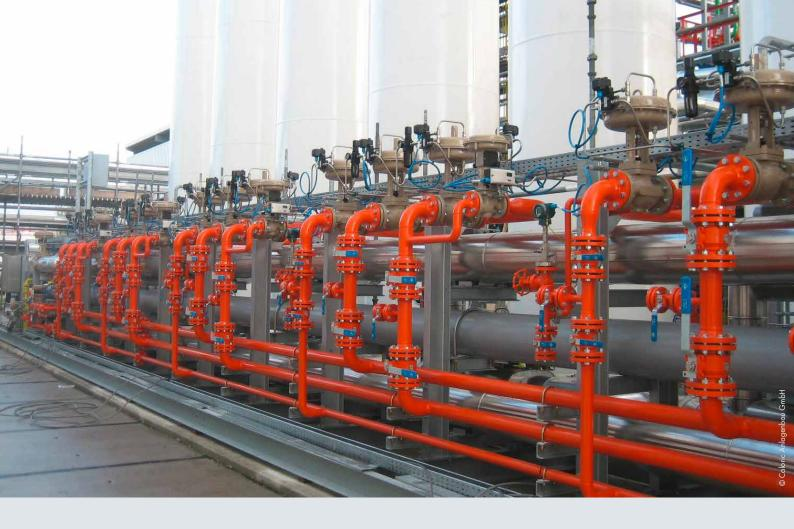
absorbents containing carbon (e.g. activated carbon or carbon molecular sieves) and oxide absorbents (e.g. zeolite) are used. The purity of the absorbed gas not only depends on the adsorbent used. The temperature and pressure during the process are important as well. As a result, the control valves used also contribute considerably to the quality of the end product.
